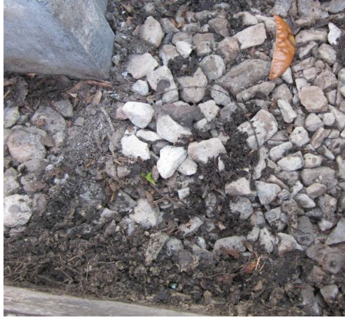
Figure 21. Sediment penetration into the storage gallery (a) Under paver blocks (b) Gravel layers
