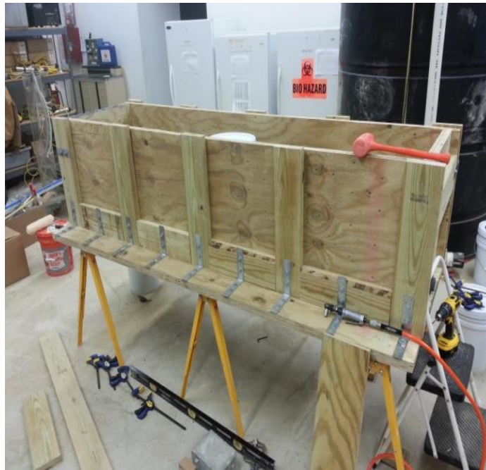
Figure 15. Structure of the flume (a) Surface preparation (b) Edge construction
