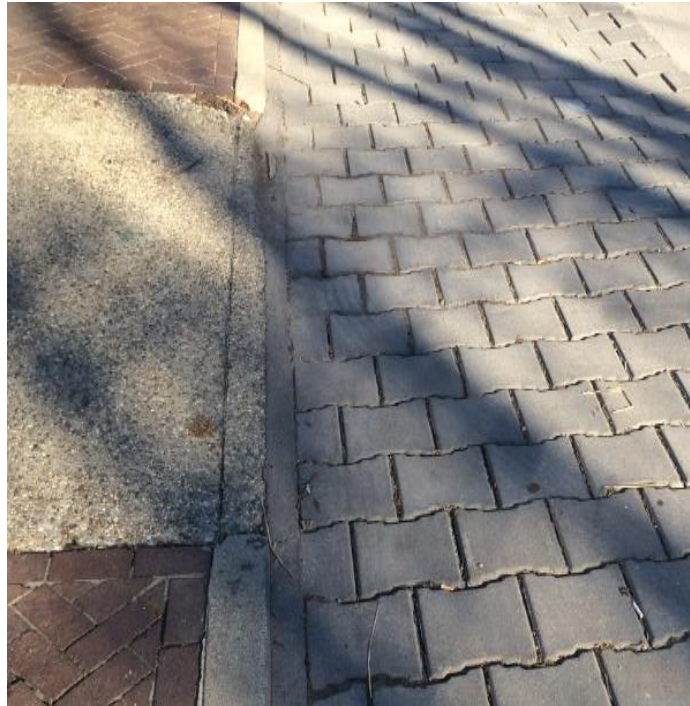
Figure 20. PICP 19H (a) Upgradient edge (b) Curb Condition
